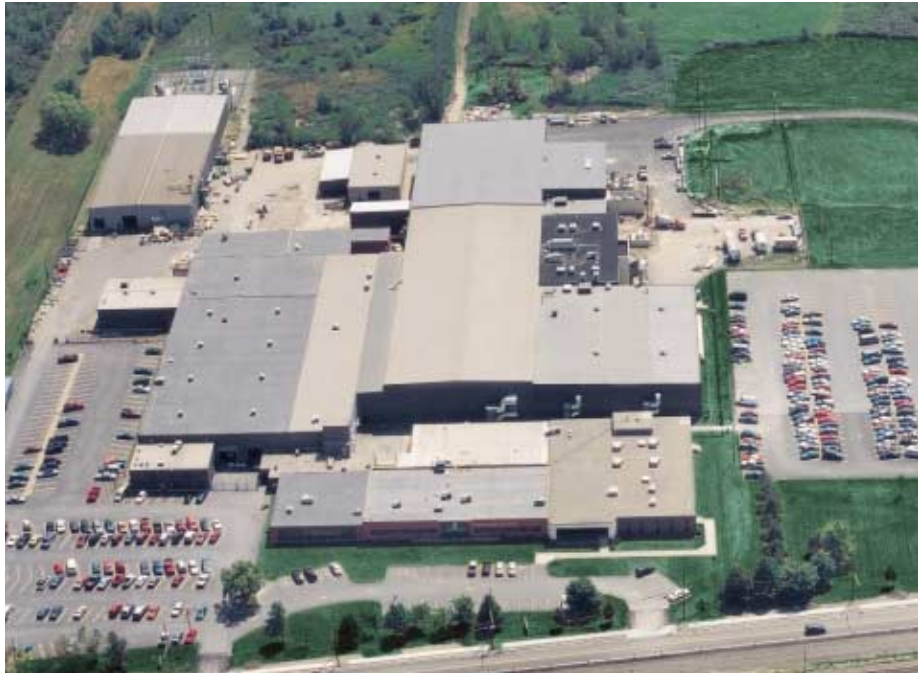
Fully integrated manufacturing facilities located in Buffalo, New York, USA are dedicated entirely to centrifugal compressors.
